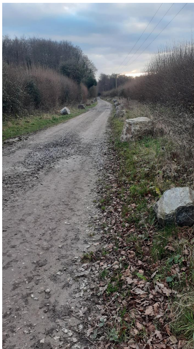
Chute BY35 - SW of Gammons Farm
